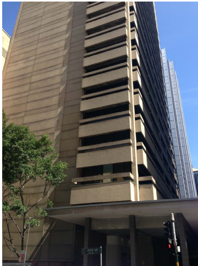
Figure 4: The eastern facade of the 1965 building
